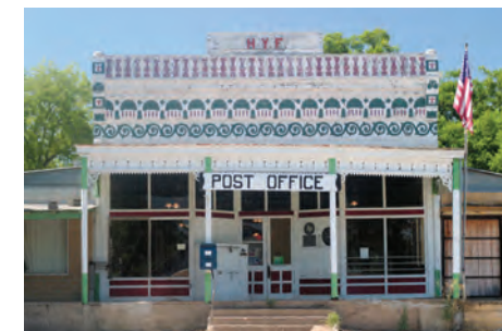
Hye Post Office, June 2005. All photos taken by Mike Francis
